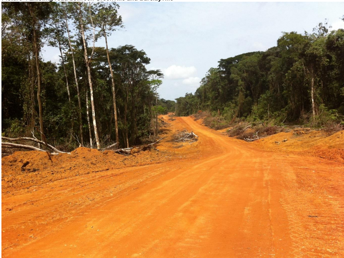
Picture 4 Existing road between Greenville and Barclayville
