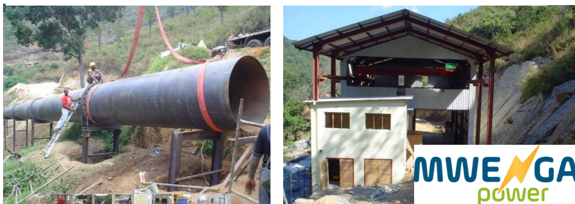
Figure 4.4.2 Mwenga hydro power plant (source: Rift Valley Energy Ltd / EU)
