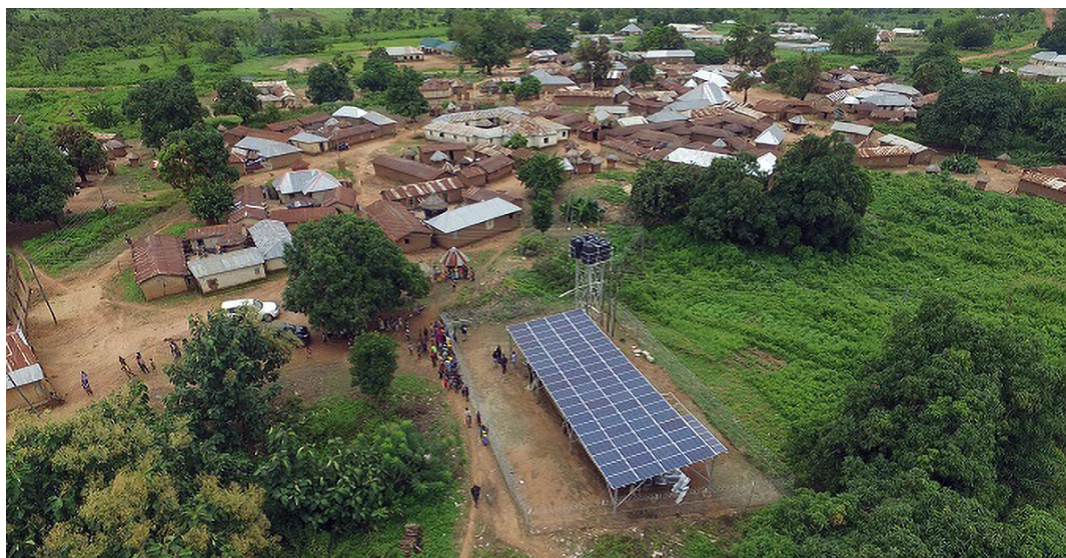
Havenhill Synergy Kigbe Solar Mini- Grid, Nigeria
