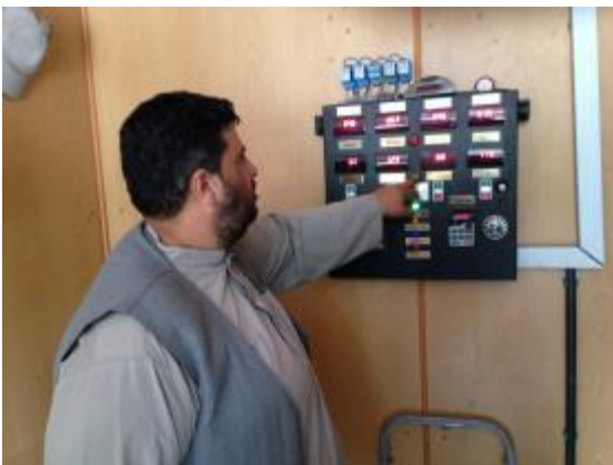
Central pump monitoring unit (self-made)
