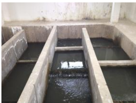
The aeration galleries of the treatment plant
