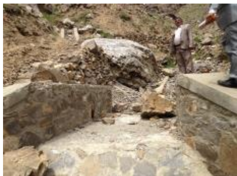
Spring protection and masonry cladding
