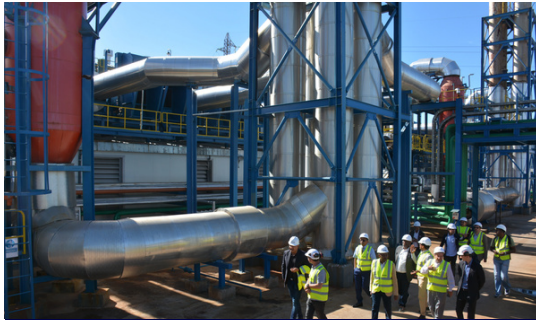
A power plant producing energy from bagasse in La Réunion (2018)
