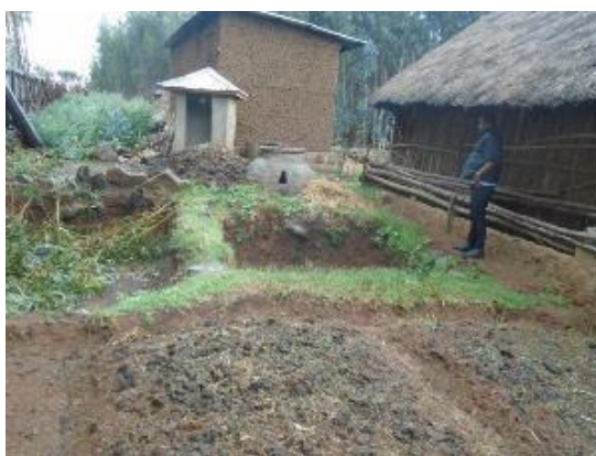
Figure 52 - Accumulation of bio-slurry around the bio-digester (Oromia_ North Shewa_ Grar Jarso_ Kotche Year 3_ Jul_ 2019_ Tariku Hailu)
