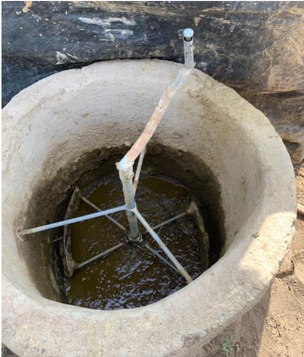
Exhibit 13. Dung water mixer (Bio-digester installations in Afar region are equipped with mixer.
