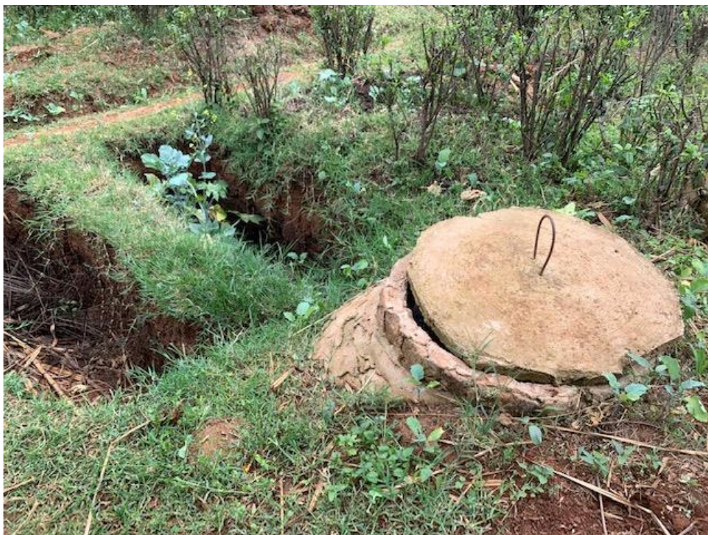
Exhibit 2. Bio-digester prone to erosion, Gozamin Woreda, East Gojjam Zone Amhara region
