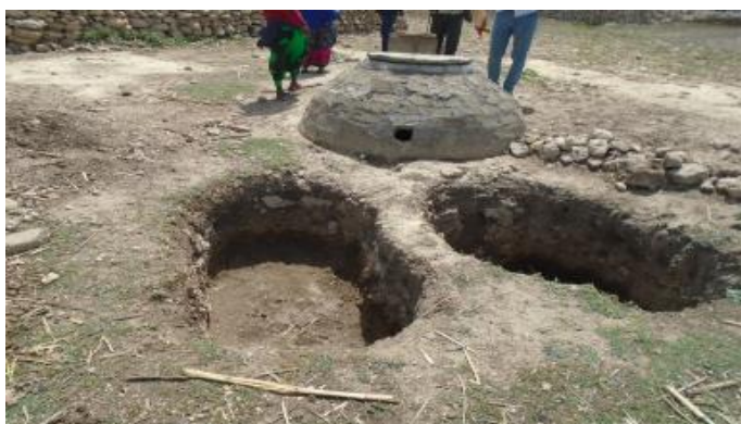
Figure 92 - Unsmoothed and high opening of the outlet of bio-digester
