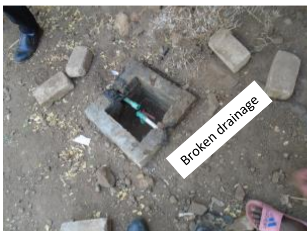
Figure 62 - Damages in bio-digester that persist in the absence of after-sales service
