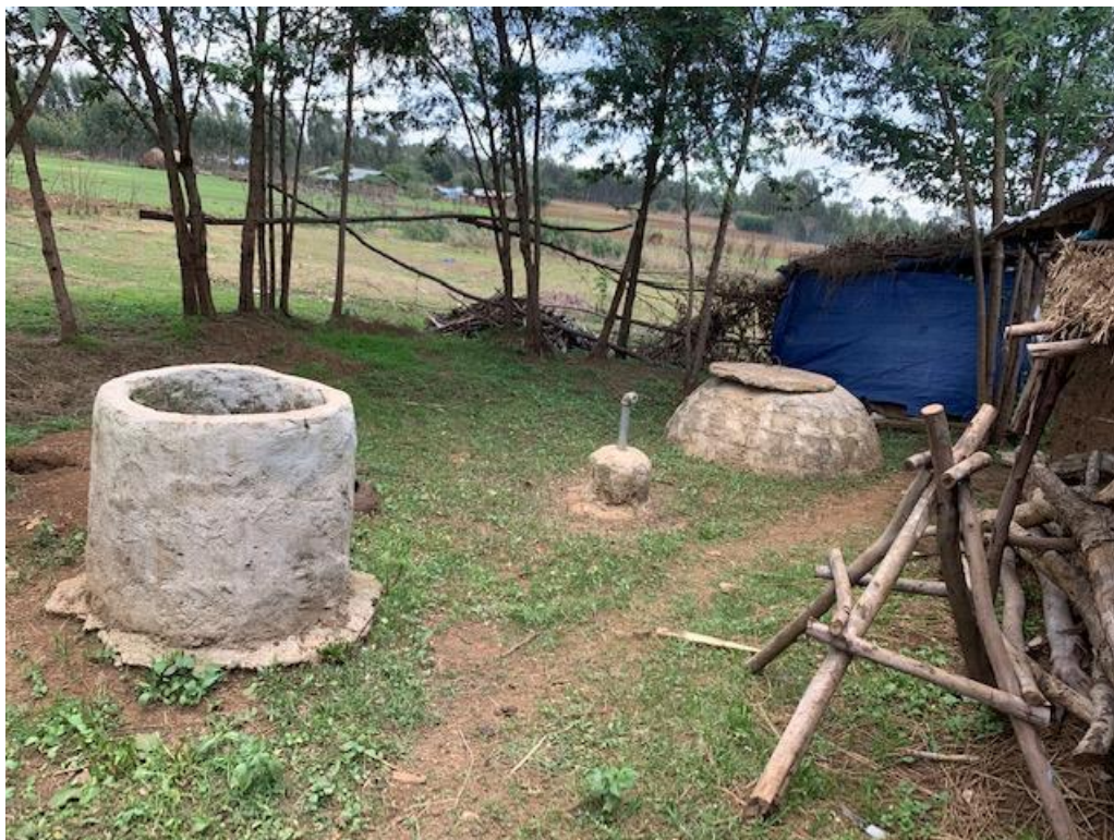
Broken pipe, Dangla Zurya, Awi Zone, Amhara region
