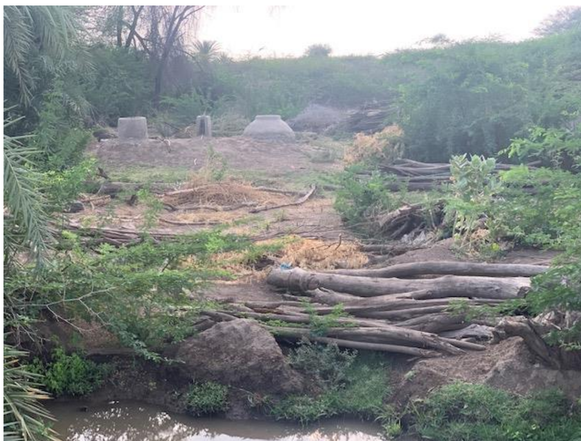
Exhibit 12. Abandoned Bio-digester due to flooding (Overflow of the Awash river). Assayita Woreda, Zone 1, Afar Region
