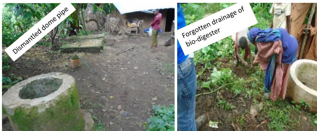
Figure 48 - Dismantled dome pipe (left) and forgotten drainage of bio-digester (right).
