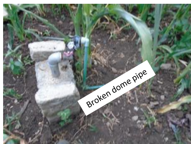
Figure 62 - Damages in bio-digester that persist in the absence of after-sales service
