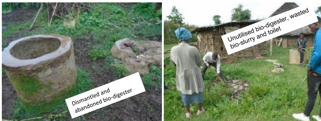
Figure 47 - Dismantled (left) and un-utilised bio-digesters (right).
