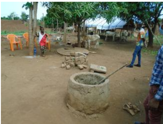
Figure 31 - Dismantled turret cover. (Gambella_Anywaa_Abobo_Mender 8 GM AB 8 Year 3_2019 Deneke Tesfaye)
