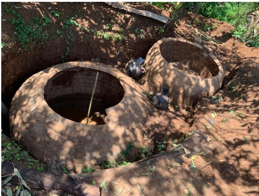
Sinking Bio-digester, Gozamin Woreda, East Gojjam Zone Amhara region
