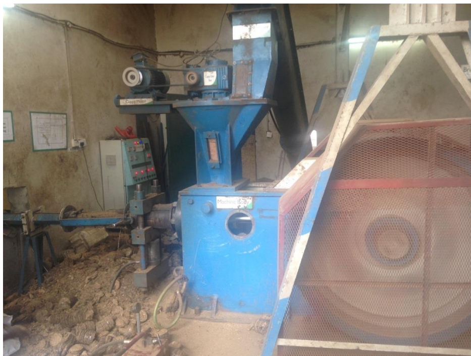
Figure D1: A motor at Lean Energy's briquetting factory in Kiambu. The briquette extrusion system can be seen on the left
