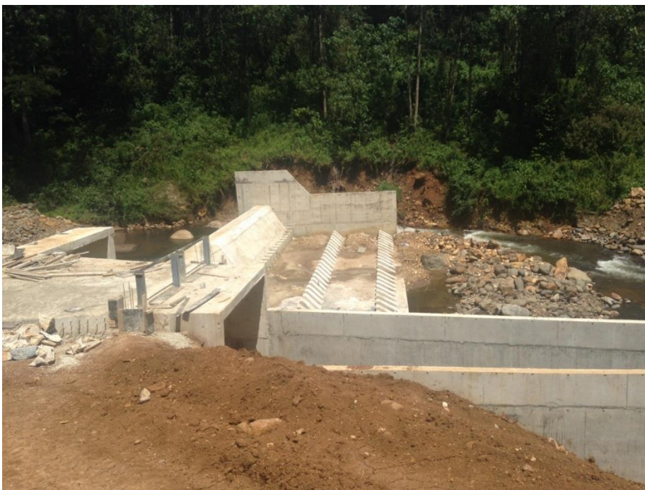
Figure C2: Intake weir under construction at Gura
