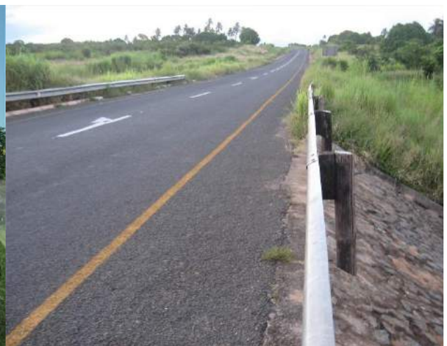
Note crash barrier at drainage structure
