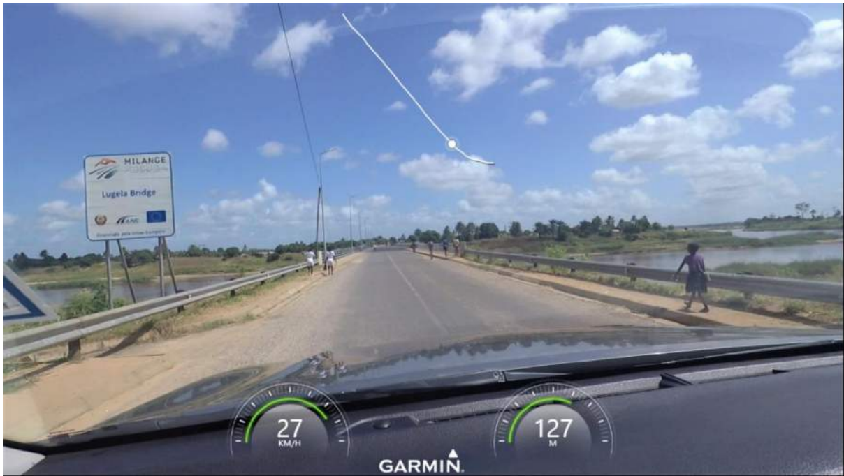
Start of the Mocuba -Lugela road at the Lugela river bridge
