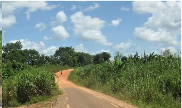
End of the road at Lugela showing the initial condition
