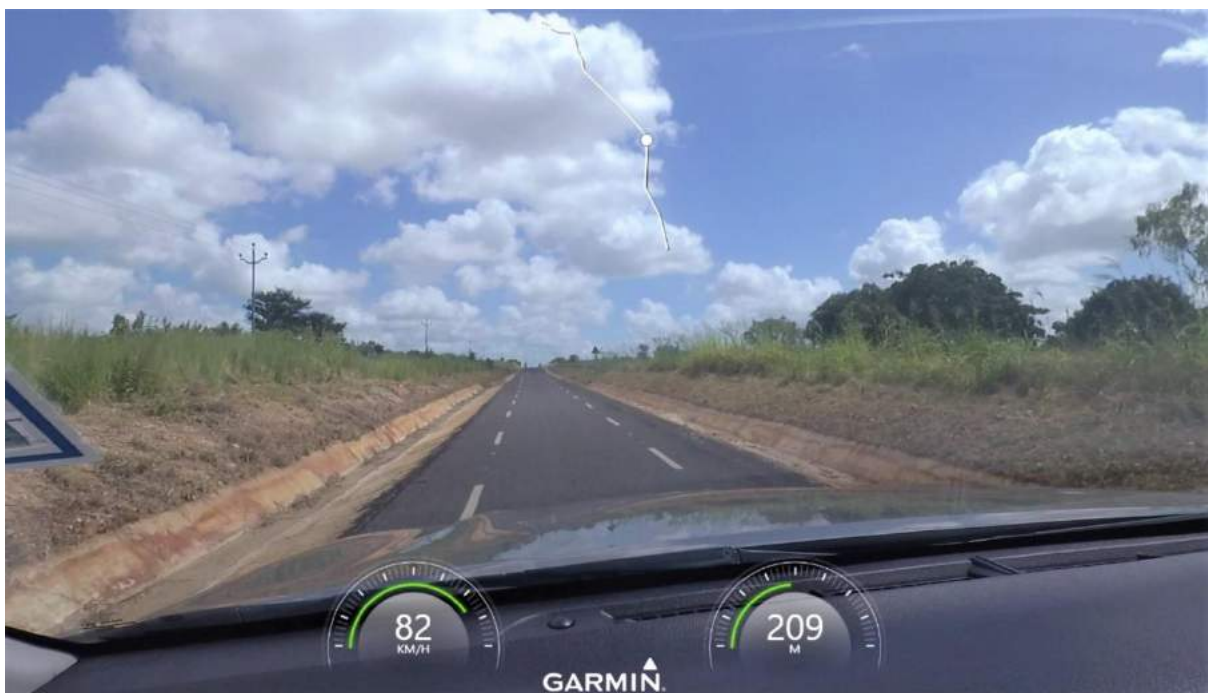
Typical section, note the concrete drainage ditches
