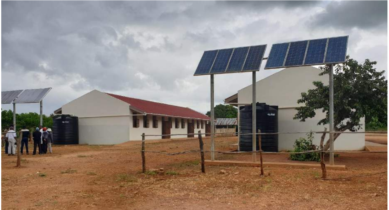
New school in Tambone. Note the watertanks that collect rain water and photo voltaic cells that provide electricity
