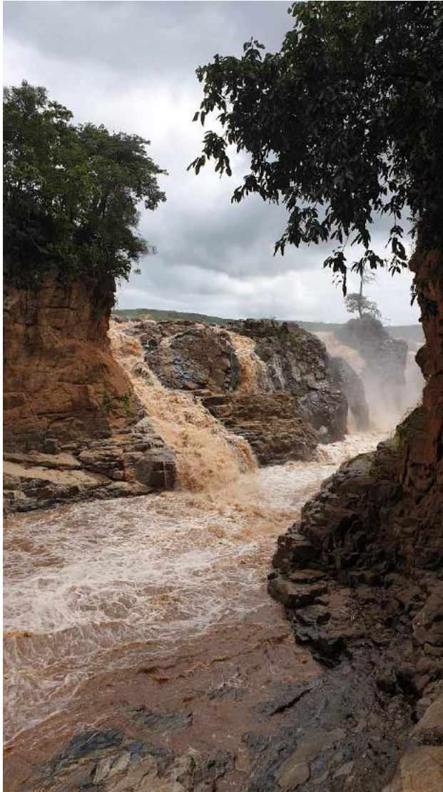
View upstream from the power station looking into the narrow canyon
