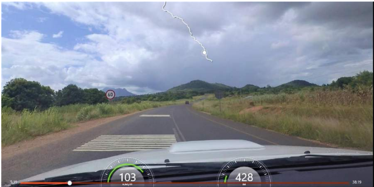
Rumble strips inform the drivers about the start of speed limits, here: 60 km/h
