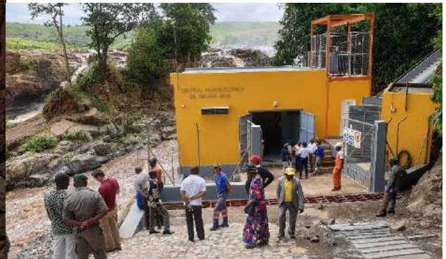
View of the powerstation
