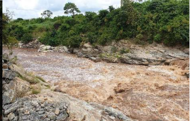
View downstream from the power station
