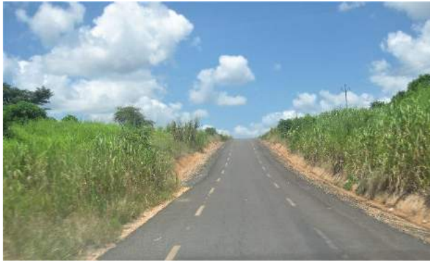
Typical section of Mocuba-Lugela road
