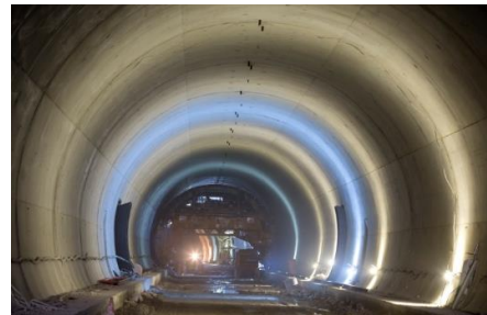
Tunnel T1 during construction
