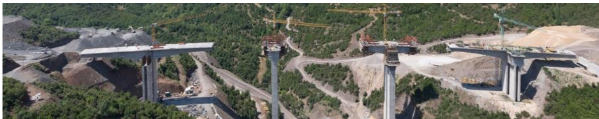
Bridge B3 during construction
