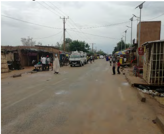
PK37- village Bonkougou- emprise insuffisante
