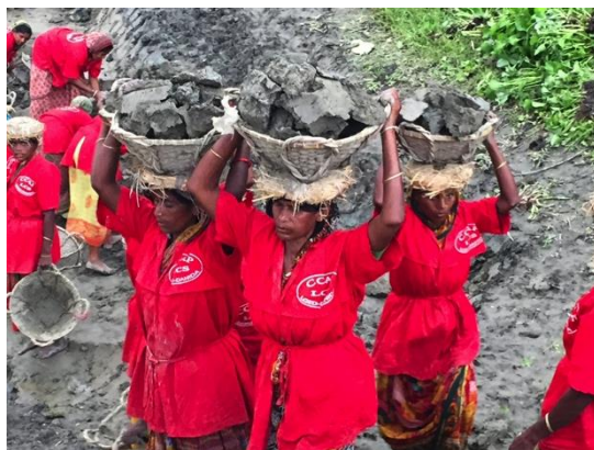
Figure 11 - Danida contracted women constructing rural roads
